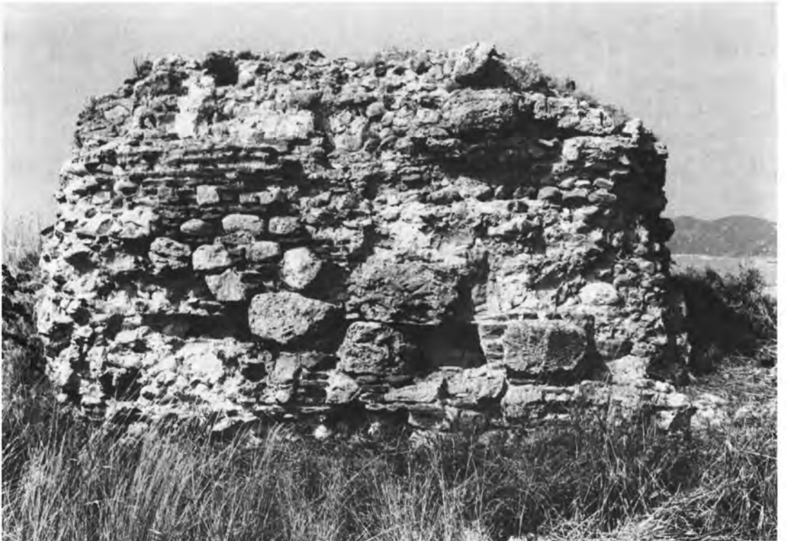
Chrysoupolis: a) West gate of Kastion dressed with antique spolia, b) The south wall, showing reuse of antique poros blocks.
