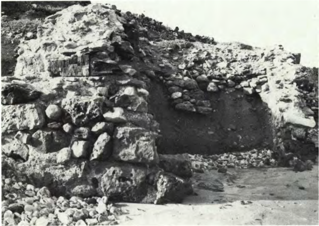
Fig. 10. The foundations of a Roman building
